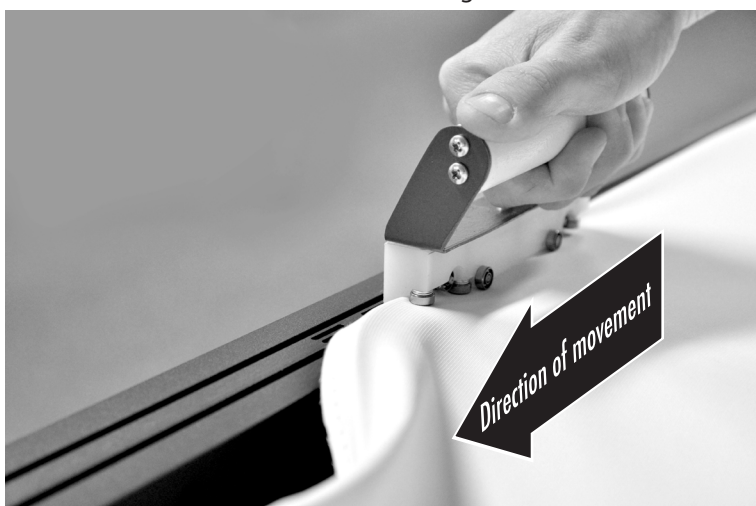
Front view of installing fabric with tool
